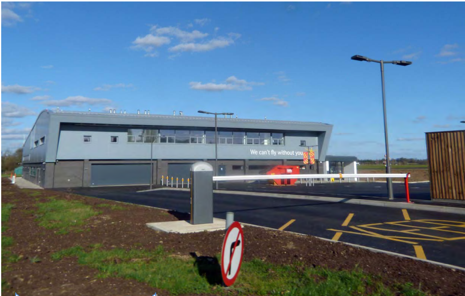
The Squadron/AeroLegends are refurbishing its old and rusty facilities with new steel in preparation for the return of Spitfires to the former fighter station ©PAR
